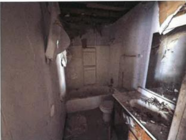
166. Building No. 17 – View of 3825 McRee Avenue bathroom.
