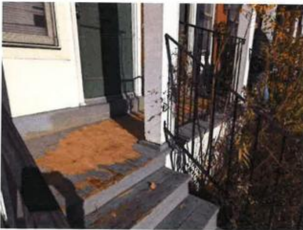
189. Building No. 21 – View of deteriorated paint at porch.
