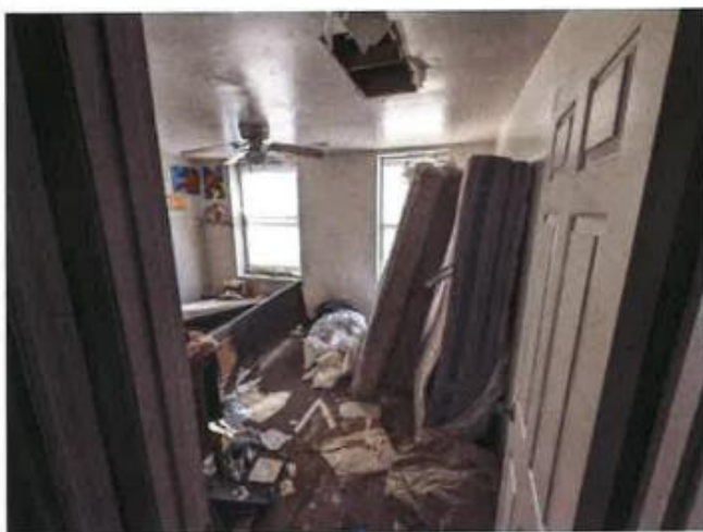
190. Building No. 22 – View of evidence of moisture intrusion at the roof of 3857 McRee Avenue.
